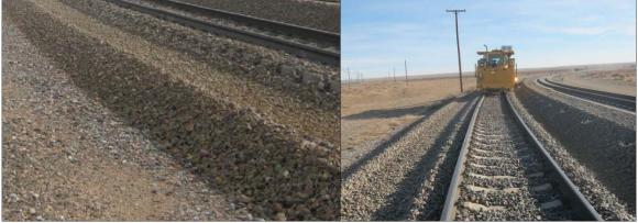
Figure 5. Shoulder Cutting to Improve Drainage
