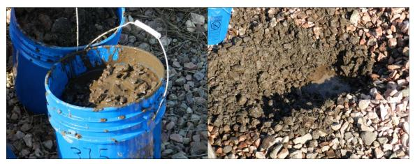
Figure 29. Example of Ballast Conditions before Ballast Shoulder Cleaning
