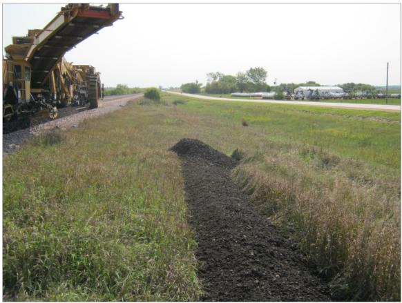
Figure 28. Disposed Waste Fines Removed by Ballast Shoulder Cleaning
