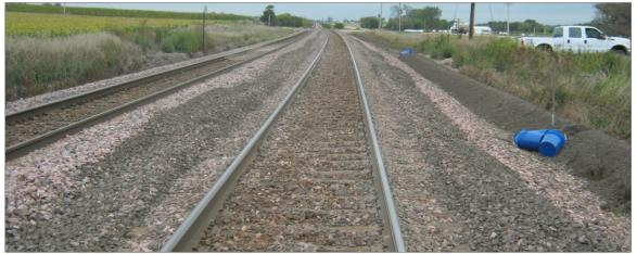
Figure 27. Test Site after Ballast Shoulder Cleaning
