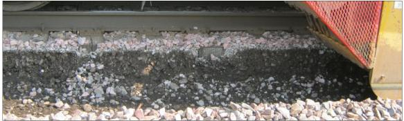
Figure 26. Exposed Ballast Section at Test Site
