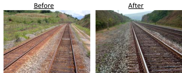
Fig. 4 (b). Steel Line – km 110 + 300
