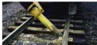
Figure 9: Nozzle rotating to 45° from vertical
