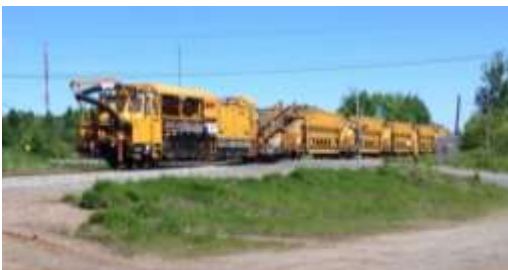
Figure [SAB6]13: Railvac Consist used on Bathurst Project
