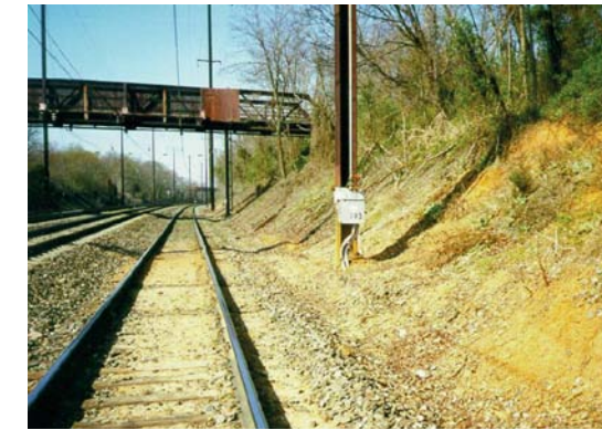
Erosion-Fouled Ditch
